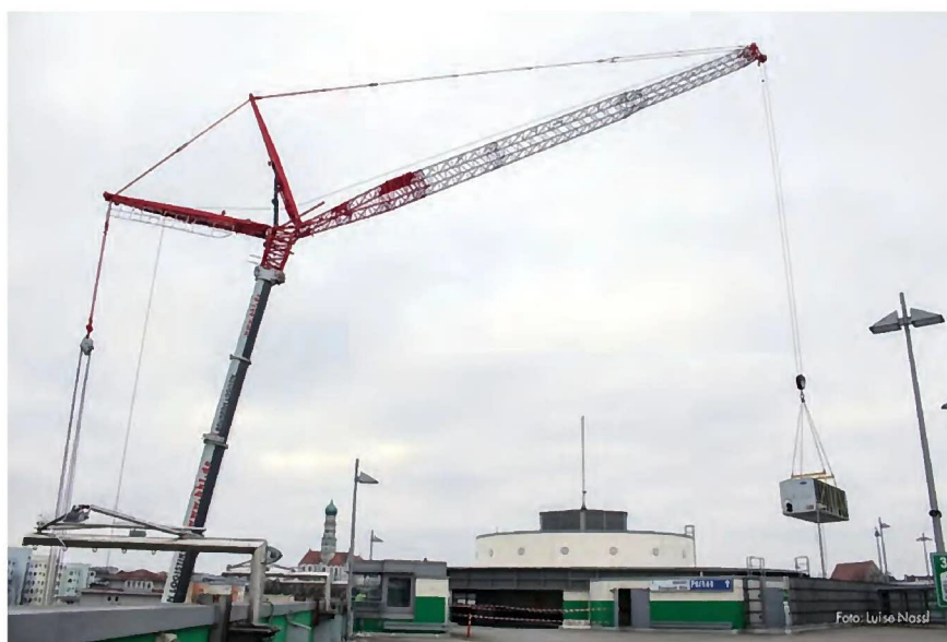
BKL in Germany stretching out one of its all terrain cranes working at the City Galerie in Germany
